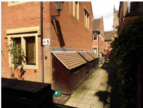
Figure 8.3.4 Locked refuse bin storage
