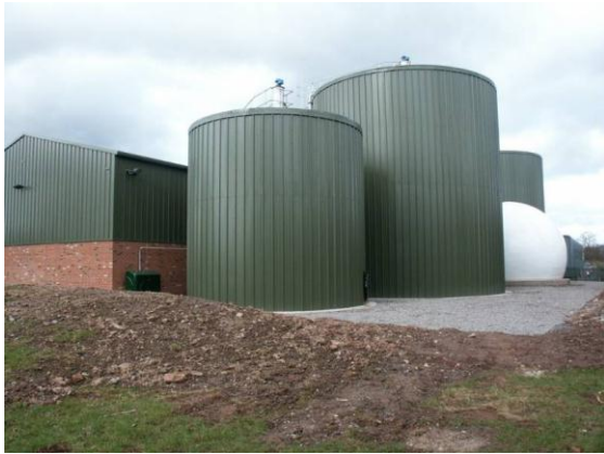
Figure 4.2.4 The Tank Compound
