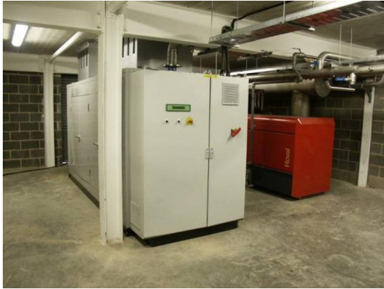
Figure 4.2.5 CHP and Standby Boilers
