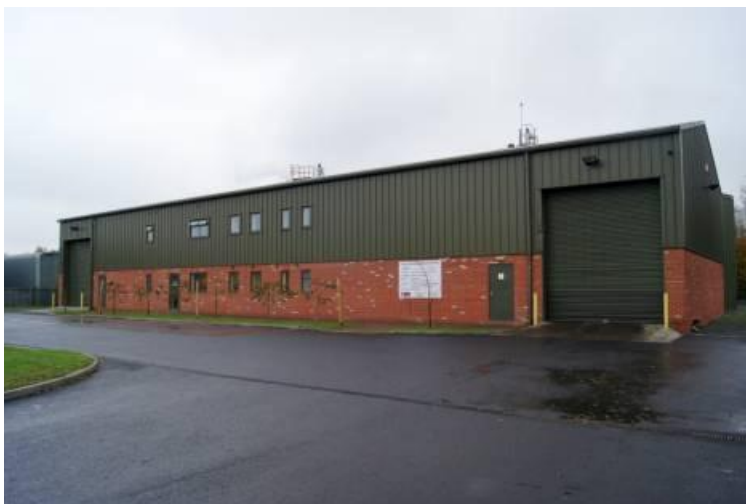
Figure 4.1.1 The South Shropshire Biowaste Digester (Biocycle)
